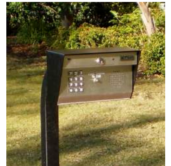
TELEPHONE ENTRY SYSTEM WITH KEYPAD
