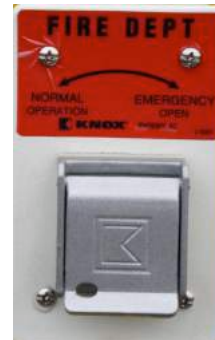
KNOX BOX EMERGENCY ACCESS SWITCH
